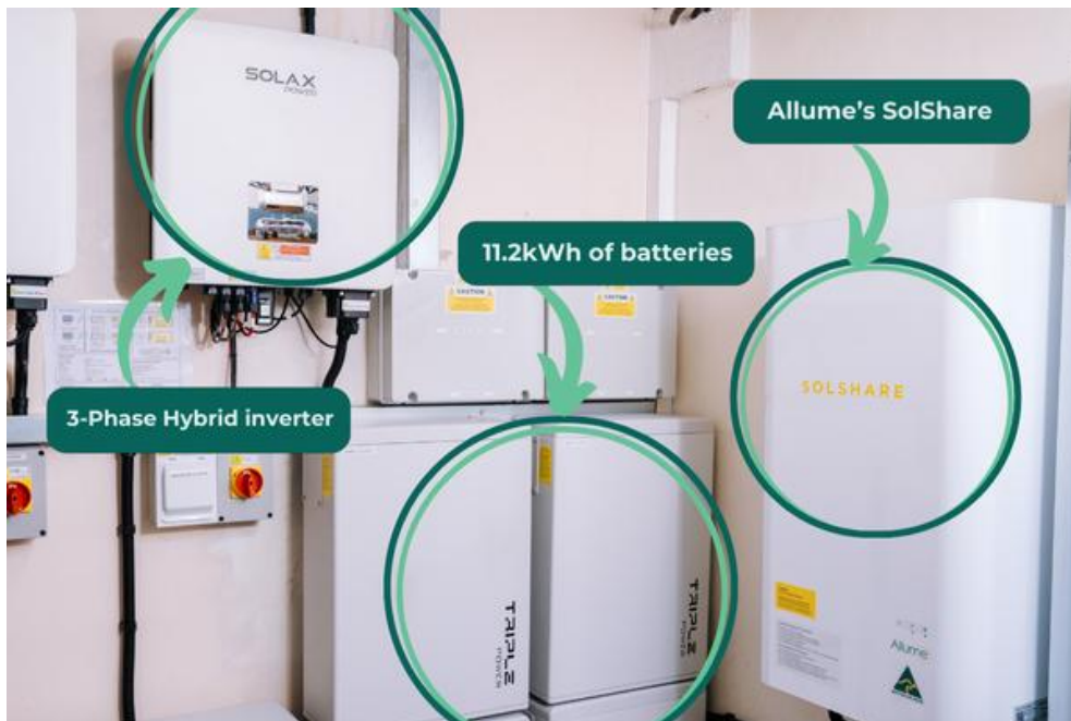
Figure 1: Showing how compact a SolShare installation is with batteries.
