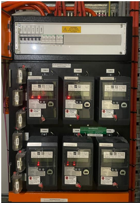
Fig 7. Meter Panel
