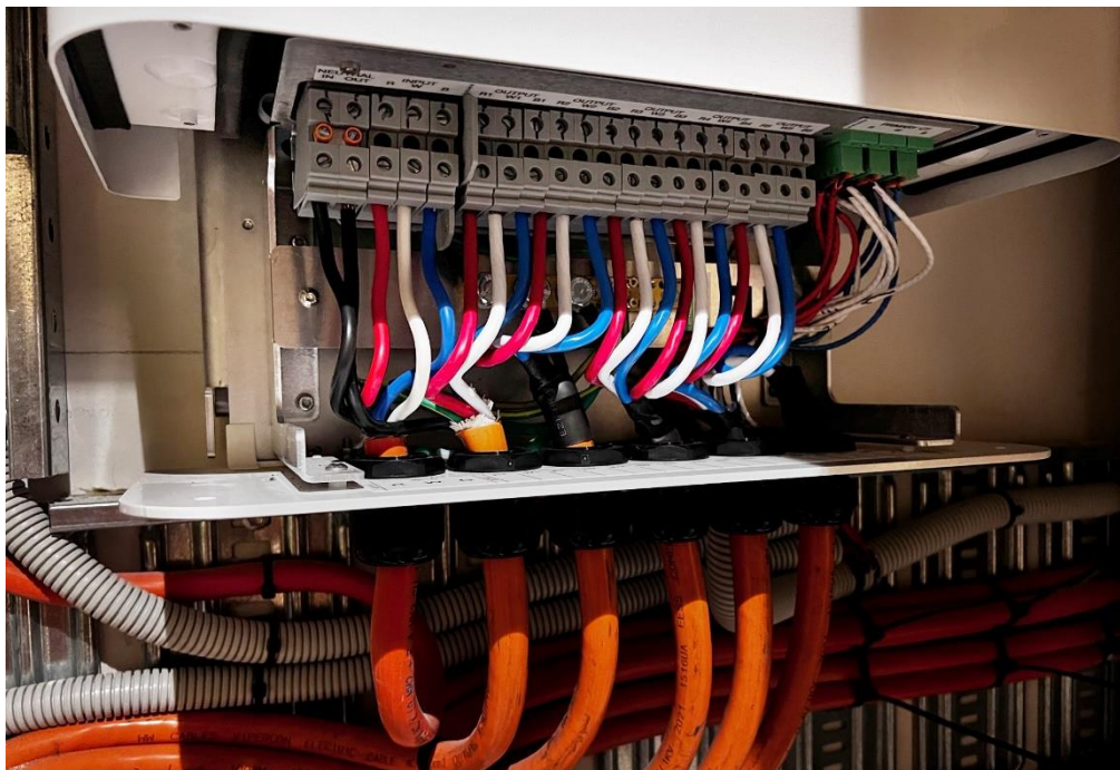
Fig 3. SolShare Installation Area
